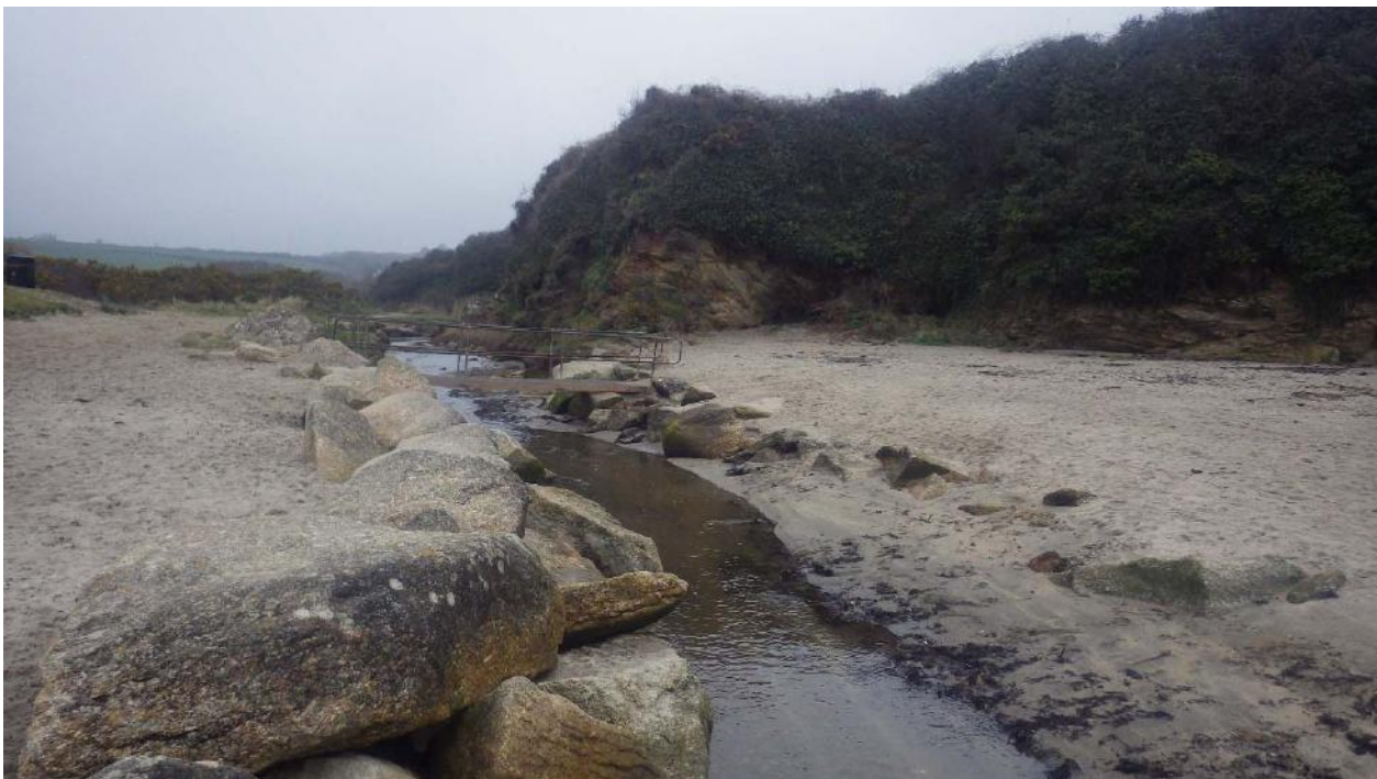
Figure 4.5 Rock boulders in Polmear stream, used to stabilise the channel (taken during site visit 12 th March 2015, above – looking south and below – looking north).
